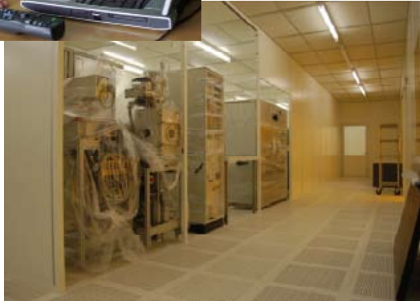
Fig.2: New clean room (clean room class 10) in the new building of the Institute for Physics
