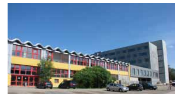
The clean room 1 of the ZfM is located in hall H next to the Weinholdbau on the Smart Systems Campus Chemnitz.
