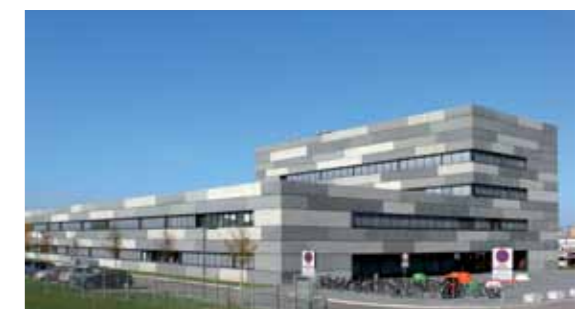
The clean room 2 of the ZfM is located in the building of the Institute of Physics, TU Chemnitz.
